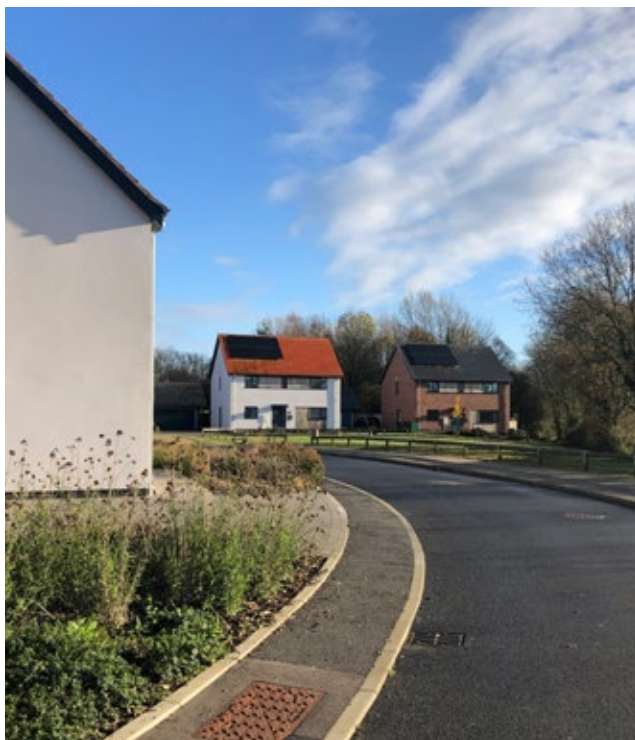
Cedar Rise development completed in 2019 at the edge of Mattishall village, south of Dereham Road. The white render facades, tiled gable roofs and spacious layout reflect the local character of Mattishall. However, the design may have been enhanced if other aspects responded to an analysis of the local context of the plot, character area and Mattishall.
