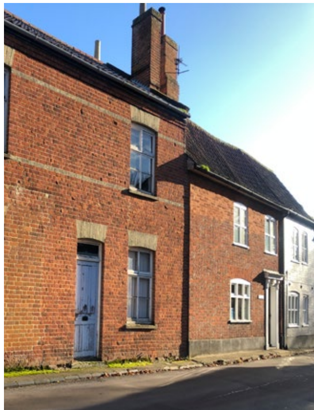
Residential buildings along Church Plain constructed with red brick walls, a slate tiled gable roofs, recessed porches, slender brick chimneys and white timber fenestration. These architectural materials and features are locally distinctive.
