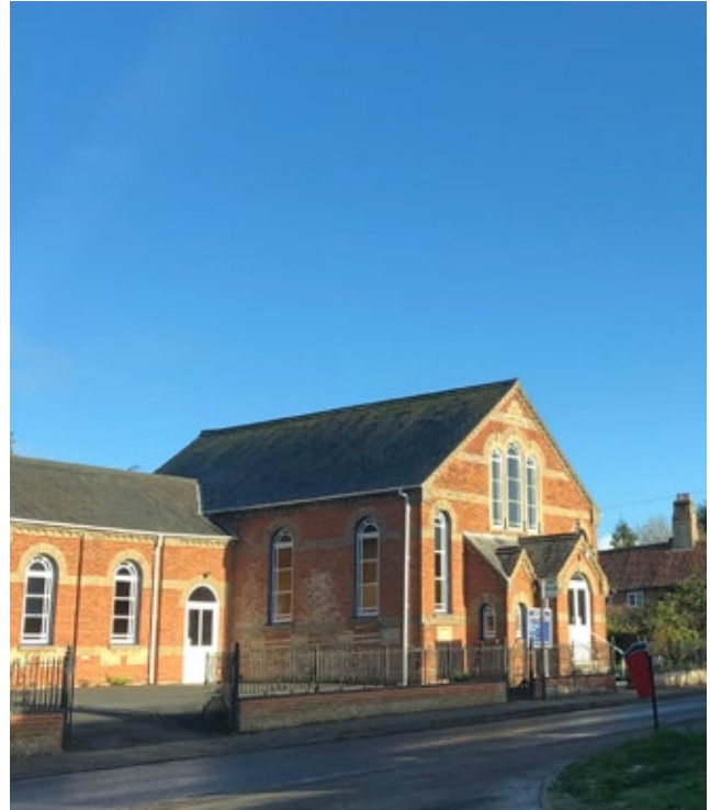
The Methodist Church building which is a key destination within the character area.
