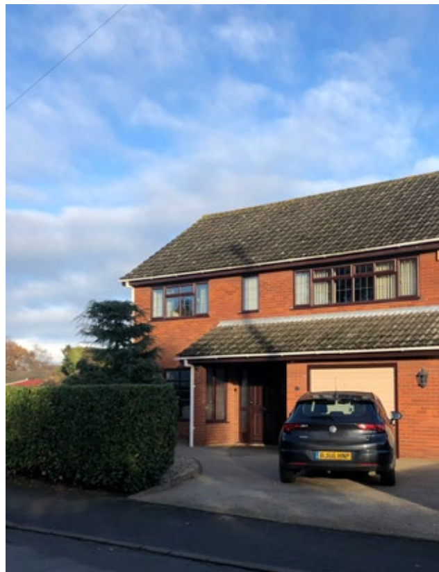
Residential building constructed during the 20th century. The red brick and tiled roof are locally distinctive. The dark brown fenestration and grey colour of the tiled roof are not typical of Mattishall's historic vernacular.
