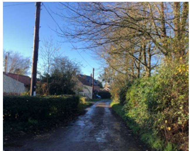
Church Lane forms the boundary of the Village Residential and Countryside Character Areas. The hedge boundary treatments that conceal buildings from the road are appropriate for the agricultural character of the settlement edge.
