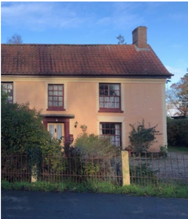
45 Dereham Road, a Grade II listed residential building. The architectural materials, colours and features are a unique architectural example within Mattishall.
