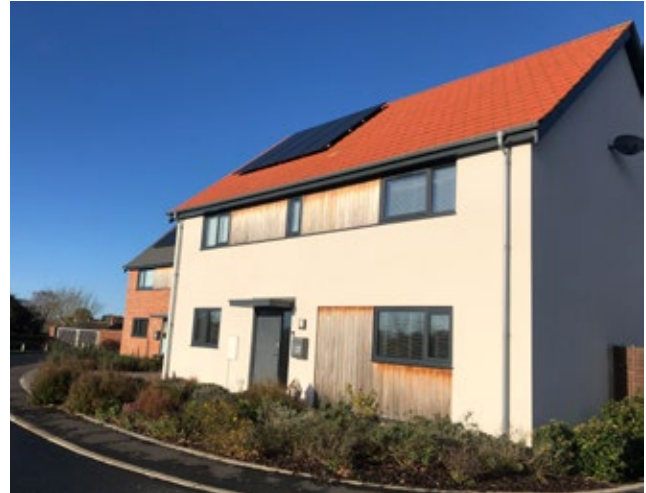
Cedar rise housing development.
